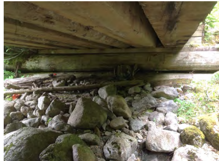
Right Bank Abutment when facing downstream
