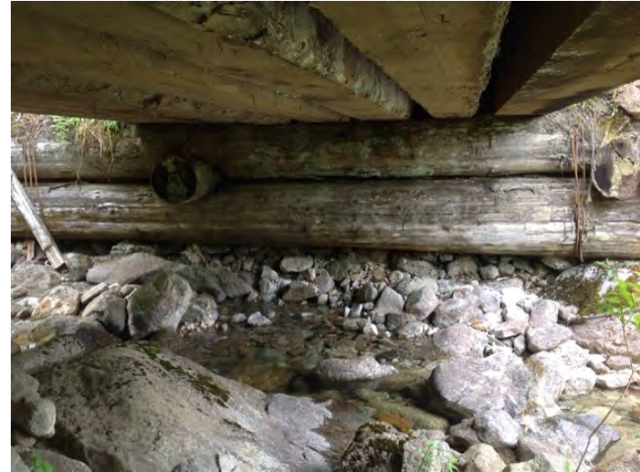
Left Bank Abutment when facing downstream
